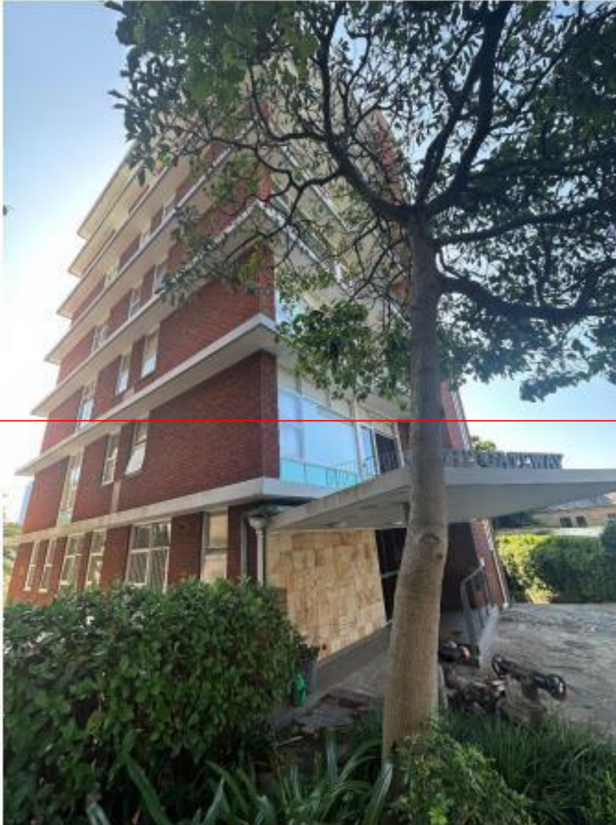
Figure 4. Gateway, 3 Wylde Street. Source: GML Heritage, 2024.
